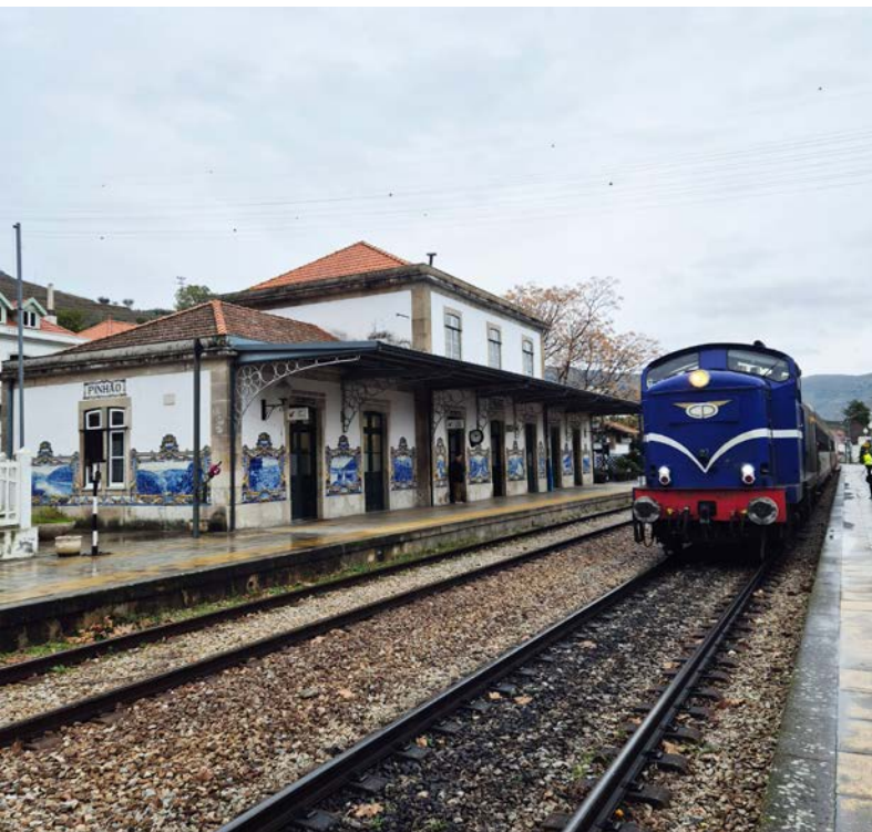
Figure 19: Pinhão station and its famous tiles. Source: Authors
