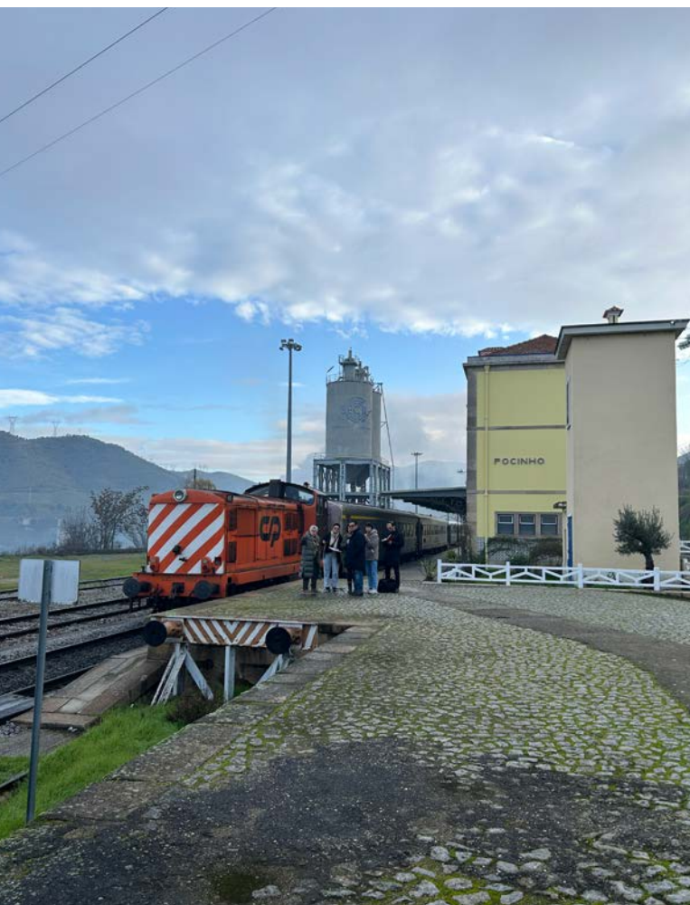
Figure 13: Pocinho station and its protected tiles. Source: Authors
