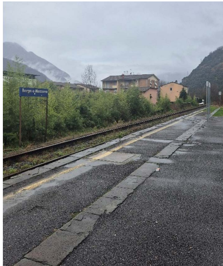
Figure 31: Borgo a Mozzano station platform. Source: Authors
